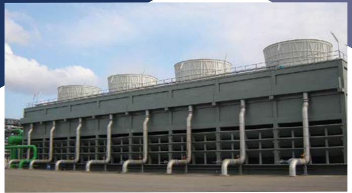
Concrete Cooling Tower in Italy
