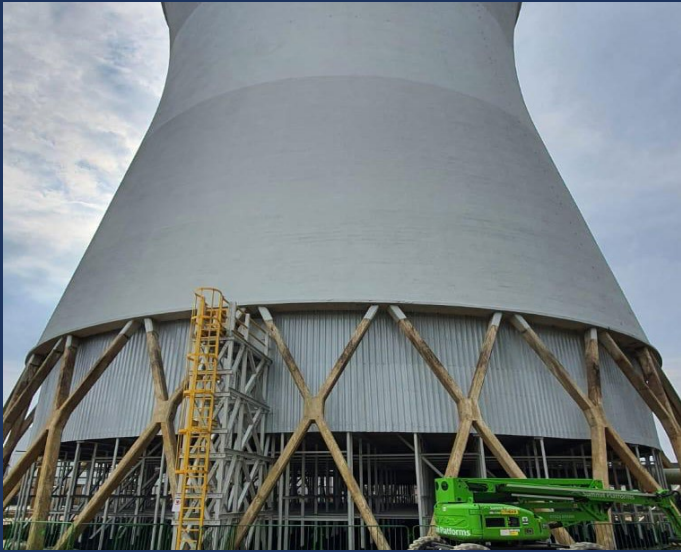
Natural Draft Cooling Tower revamping activities in UK
