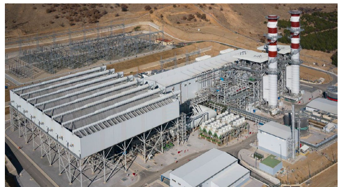
Air-Cooled Condenser and Air-Fin Cooler in Turkey
