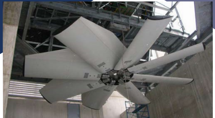
Air-Cooled Condenser installation
